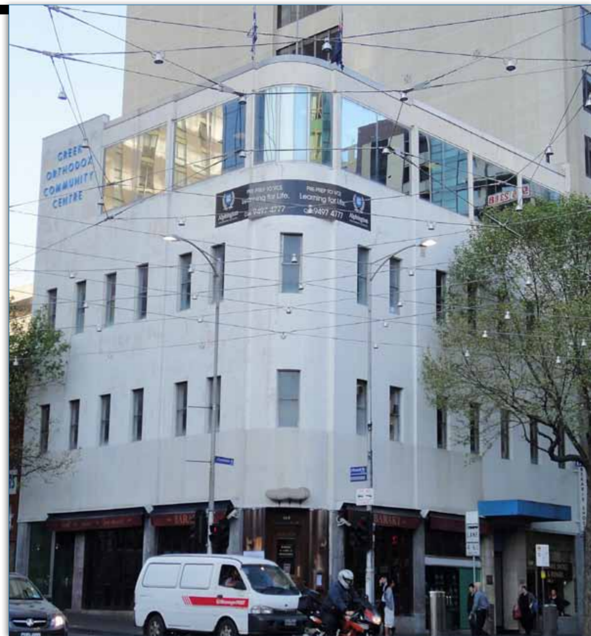
The GCM old building
